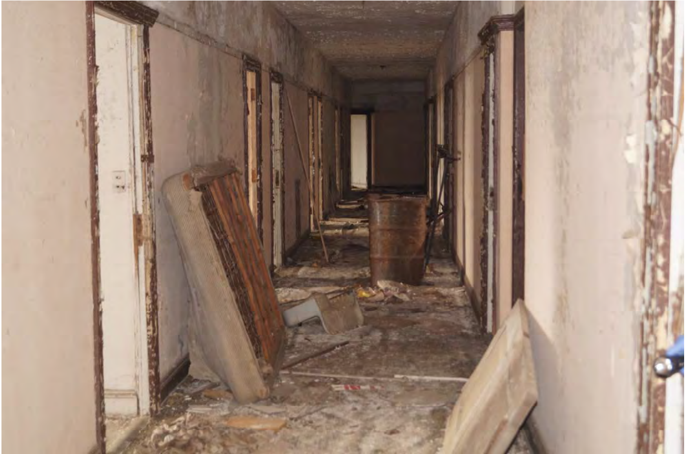
Typical Upper floor Hallway
