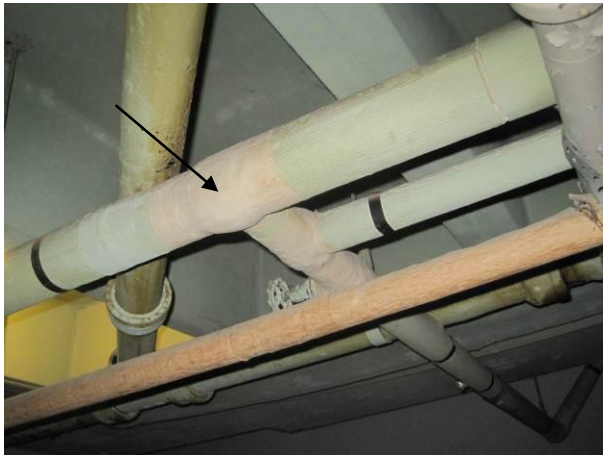
Photo #61 Asbestos-containing Thermal Fitting Insulation (White) Associated with Thermal Pipe Insulation (White, with Paper Wrap).
