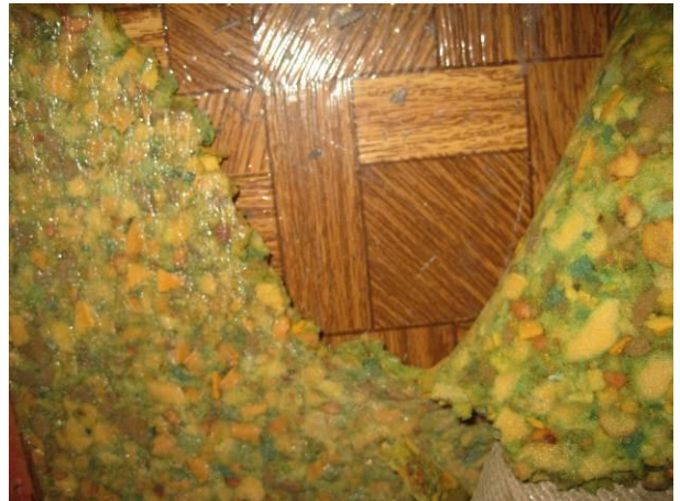
Photo #26 Asbestos-containing Resilient Sheet Flooring (Wood Pattern) with Mastic (Yellow).
