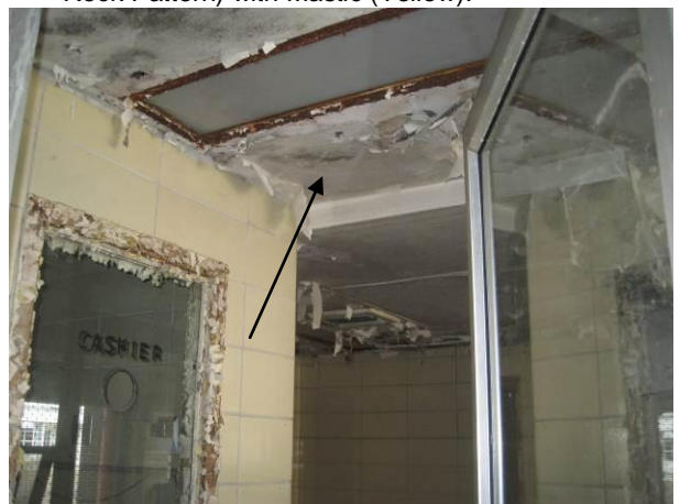
Photo #66 Asbestos-containing Wall / Ceiling Texture / Drywall / Joint Compound (White, Rough).
