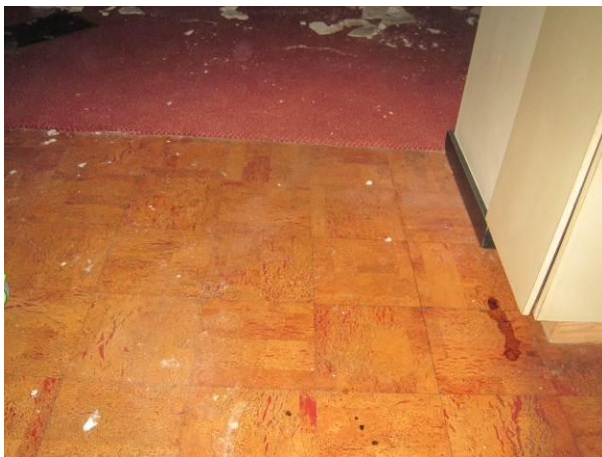
Photo #17 Asbestos-containing Mastic (Black) associated with 12" x 12" Floor Tile (Orange and Red).
