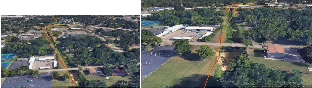
Figure 22 a and b. Aerial Views North along Projects 2 and 3.
