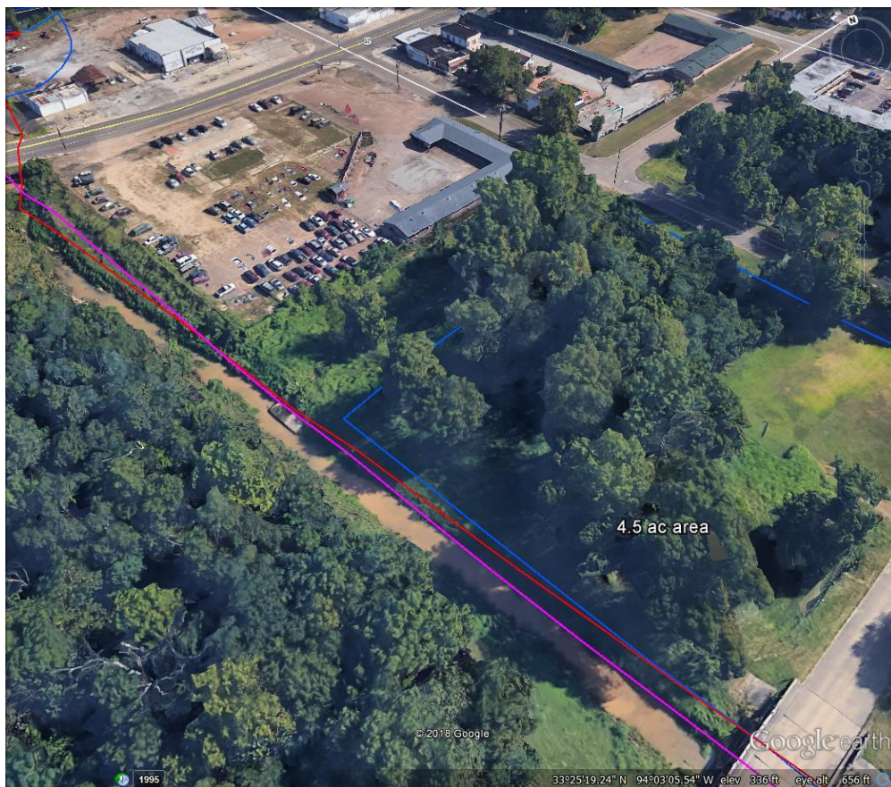
Figure 47. Aerial View of Northern End of Project 9.
