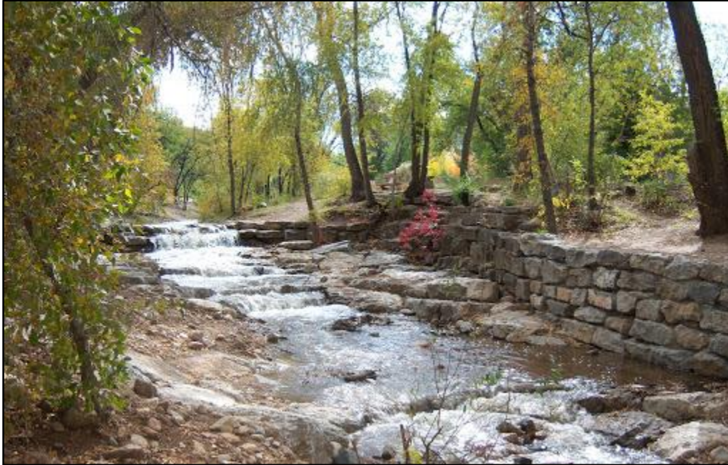
Figure 84. Patterned Colored Concrete Mimics Riffles and Pool Sequences to Naturalize.
