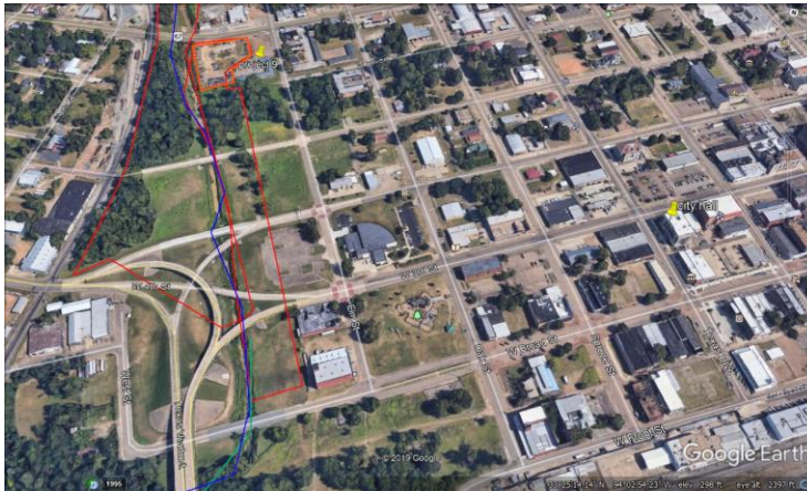
Figure 45. Aerial View Project Site 9 Showing Proximity to Downtown.
