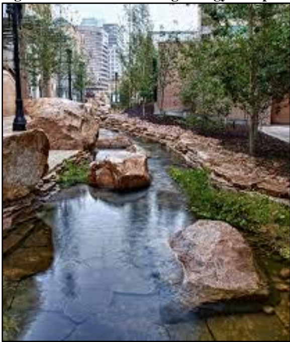
Figure 87. Artificial Boulders to Slow Flows yet Look Natural.
