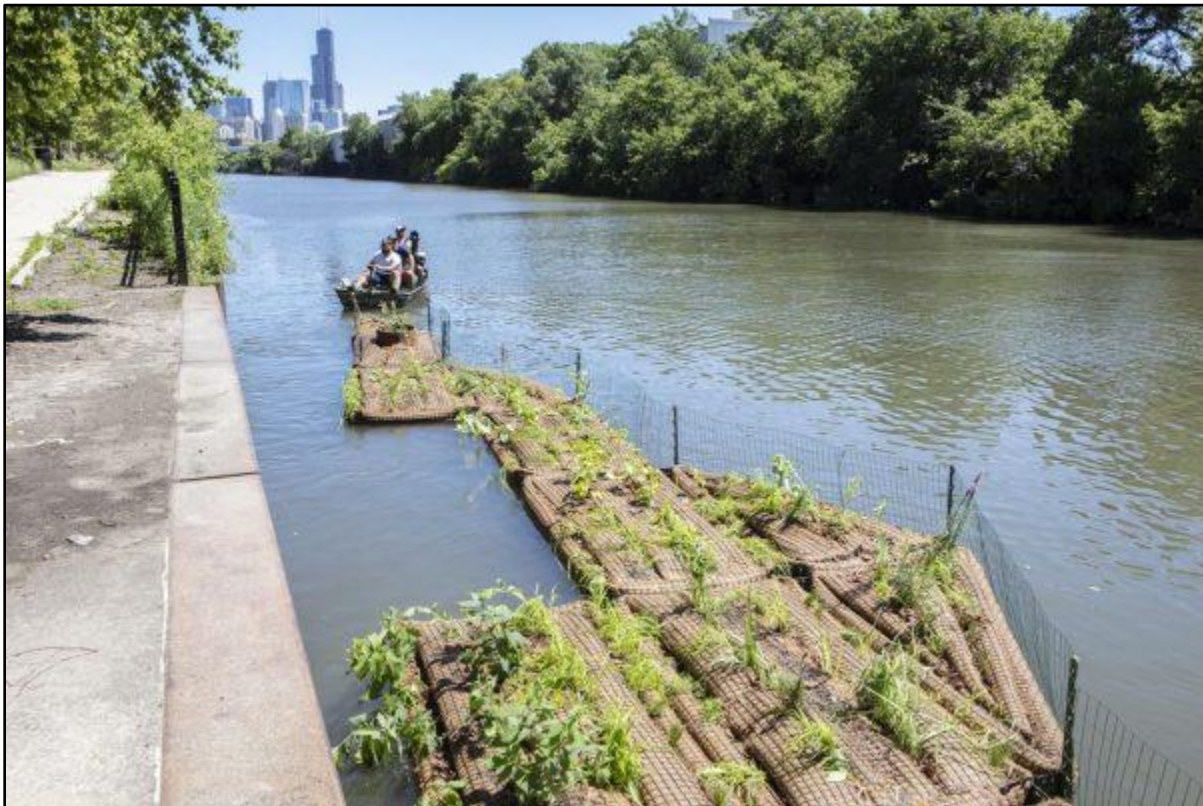
Figure 83. Floating Anchored Constructed Wetland Island in Chicago River.
