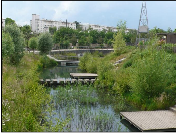
Figure 86. Dual Functioning Energy Dissipators Providing Pedestrian Stream Crossing.
